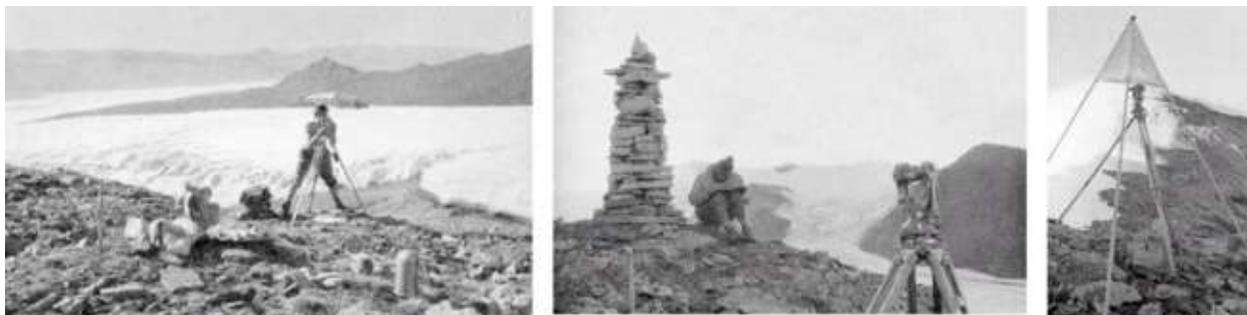
Figure 11. Wild T2 theodolite (left), stone cairns (center) and tripod signals (right).
