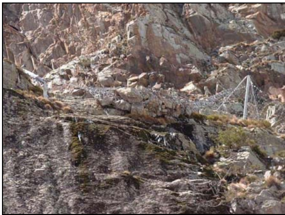
Figure 21: Picture showing mass stopped by one of the upper barriers in April 2003 event.
